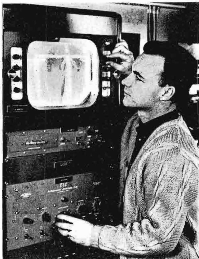
Wheelhouse control console brings in pickup from any of shipboard system's four television cameras.
