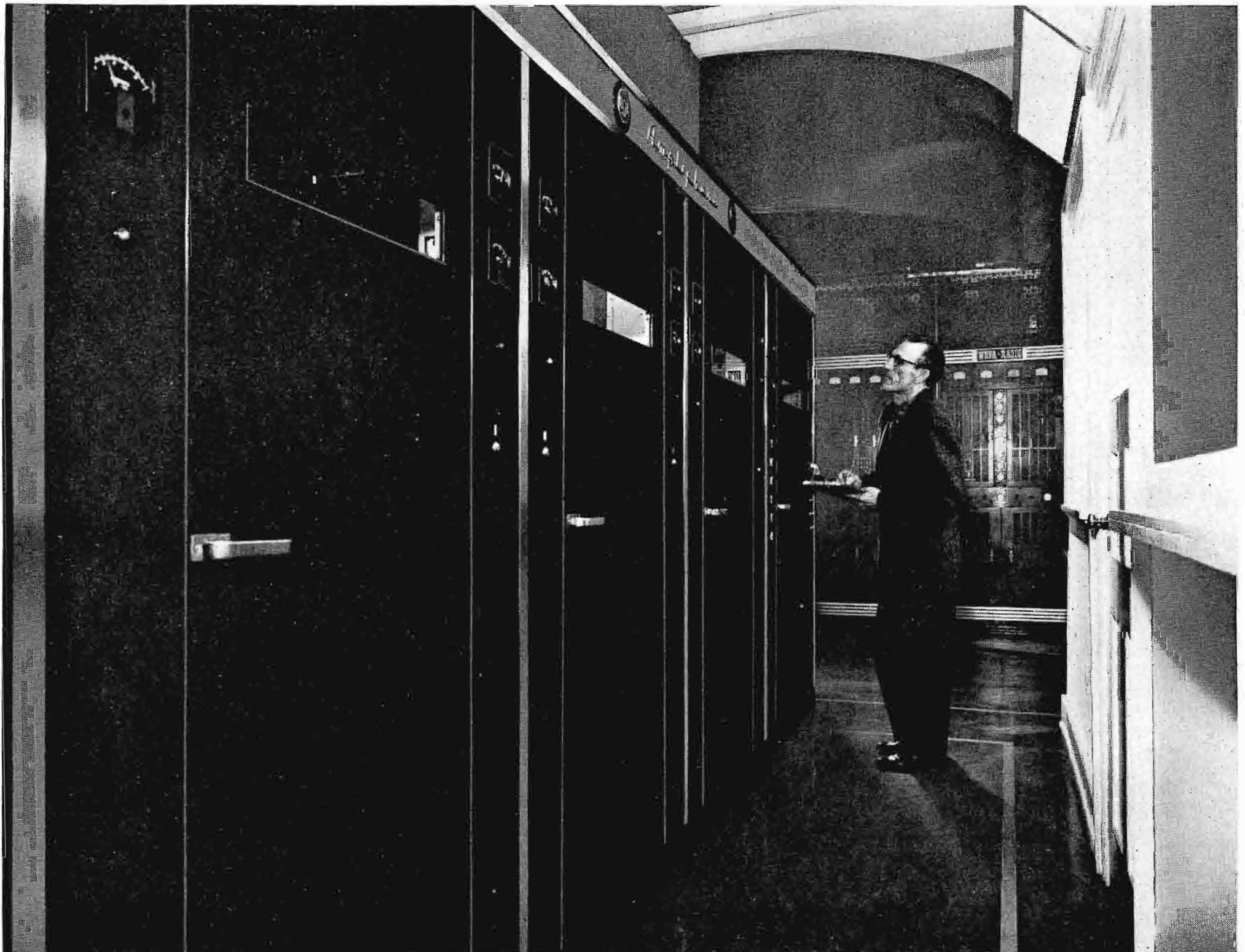
FIG. 1. A down-the-front view of the new RCA 50H with the old 50 kw transmitter in the background on the other side of the front-to-rear center corridor of the building. The exhaust duct exits through the upper half of a window
