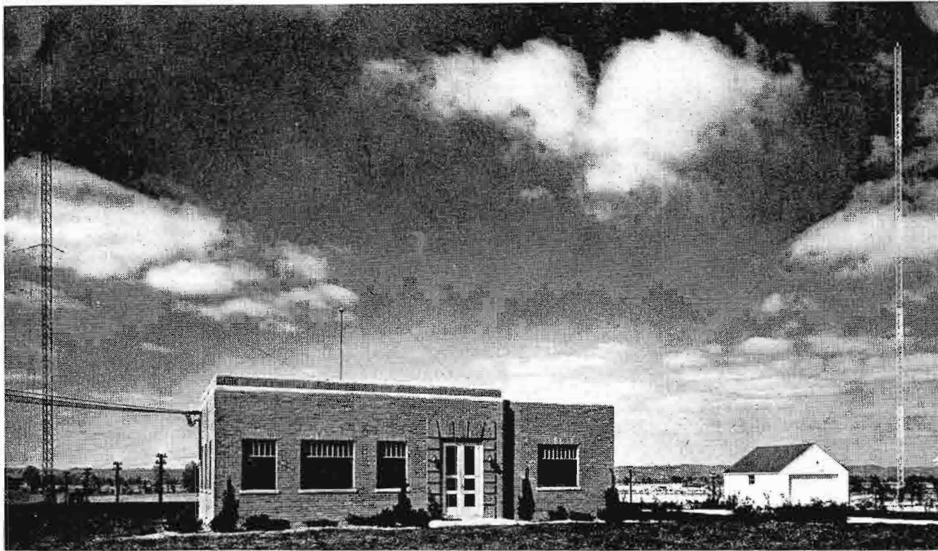
FIG. 31. AM radio transmitter building in Jeffersonville, Ind. Note 2-tower array, at right and left. For normal operation, transmitter is remotely controlled from downtown Louisville studio.
